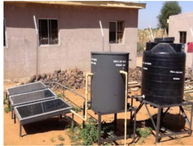
Solar Water Heater for the Health Centre
