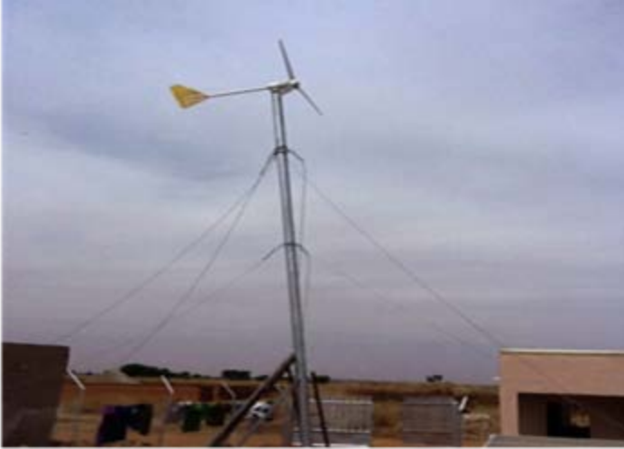
4kW Wind Power System In Integrated with 10kW Solar PV Plant (Hybrid) in Danjawa, Sokoto State , 2012
