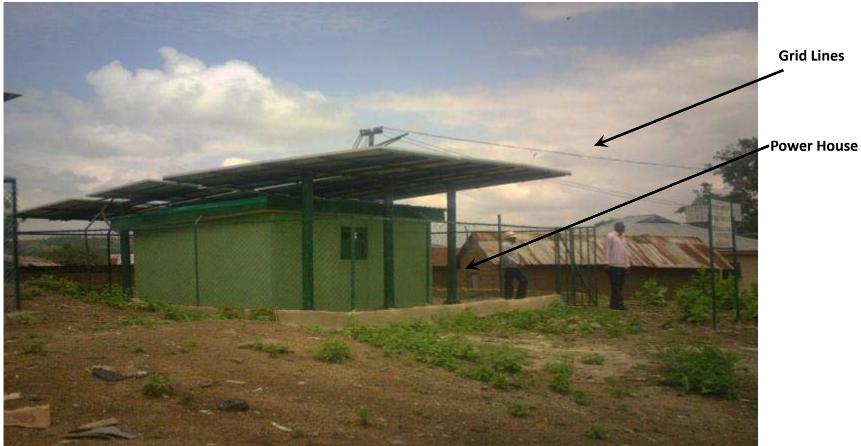
3kW Solar PV mini Grid for Electricity at Igu Community Bwari, FCT, 2012
