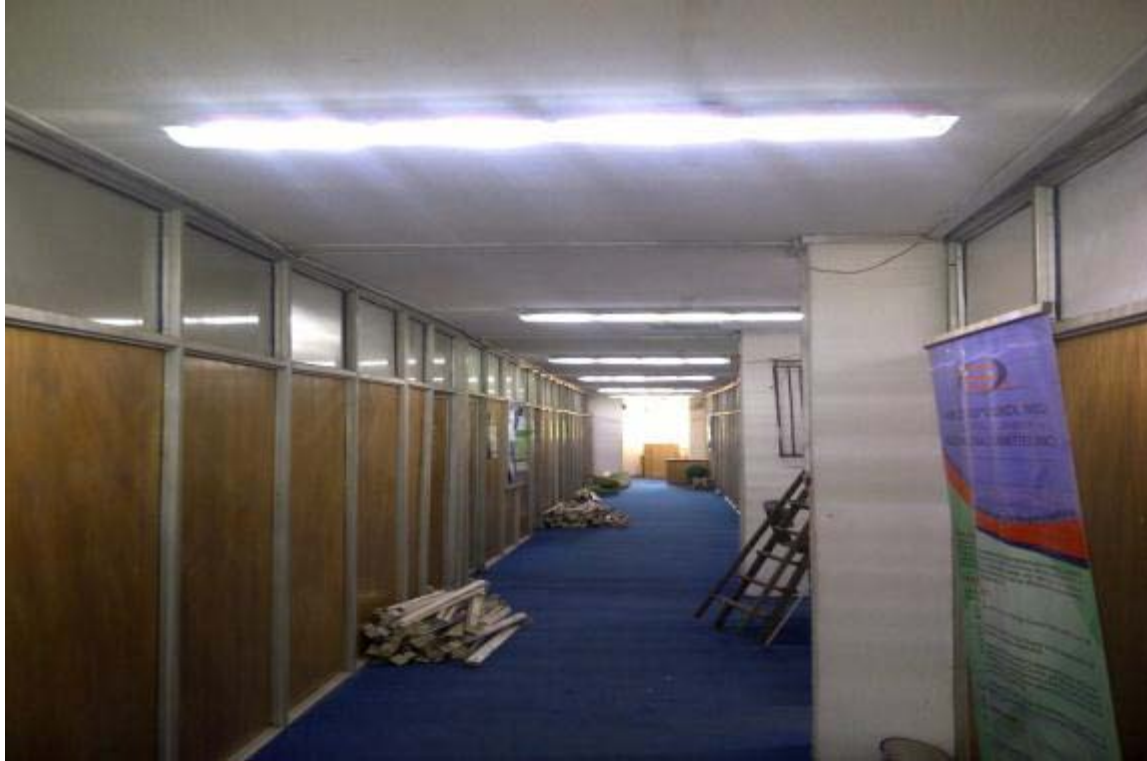
Retrofitting ECN Building with LED Lamps to half the lighting load of the building (UNDP-GEF Energy Efficiency project), 2012
