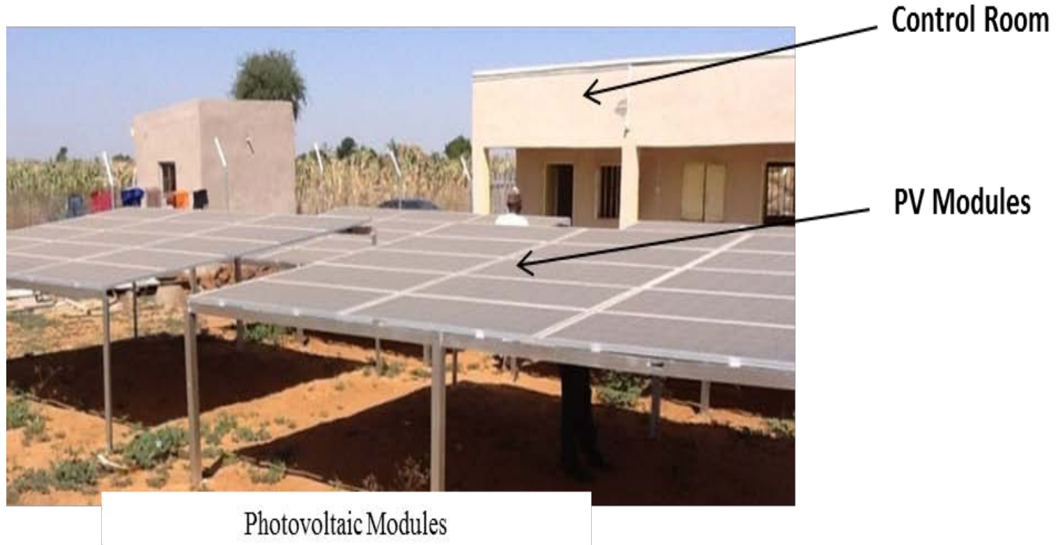
10kVA Solar PV Mini-grid in Danjawa Village, Sokoto State
