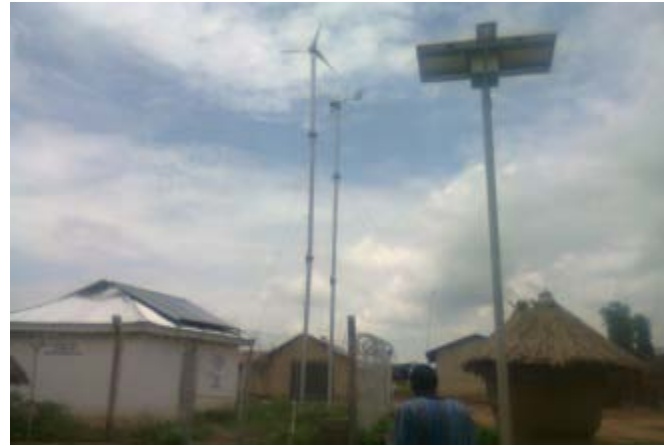
2X0.25kW Wind-Solar PV Hybrid Power System & Solar PV Streetlight at Sabon Iddo, Airport Road, Abuja, FCT, 2011
