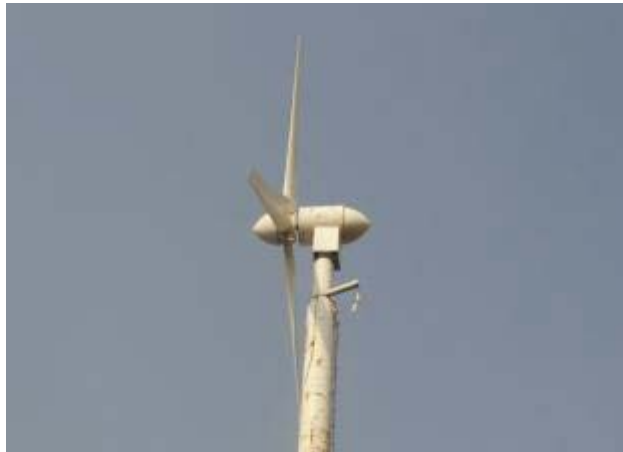
0.5kW Wind Power System for Village Electrification, at Bmuko, Dutsen Alhaji, Bwari Area Council, FCT, 2011
